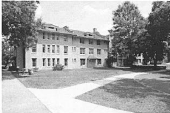
East Residence Hall at Duke University, recently renamed from Aycock Hall after a student campaign protesting the building's namesake, former North Carolina Governor Charles Aycock, a noted white supremacist. (Duke University Photography)
